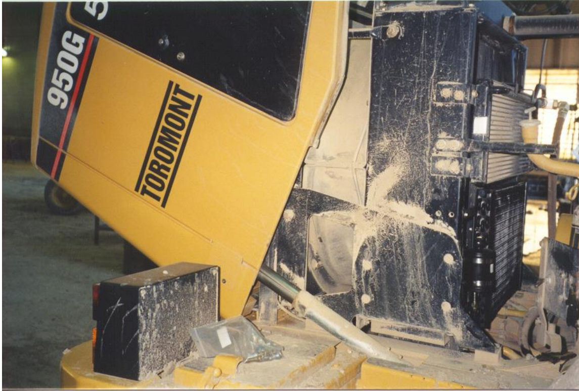
Condenser as viewed from right side.
